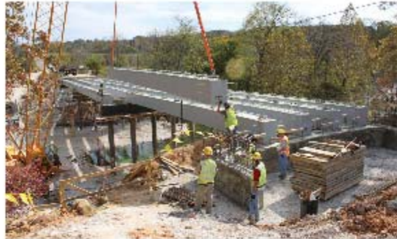
Figure 2: Erection of Hybrid-Composite Beams in Douglas County, Missouri
