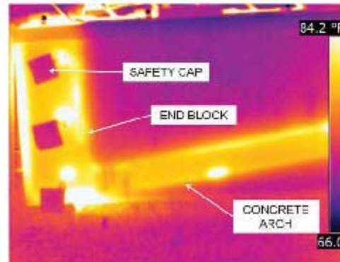
Figure 3: Thermal Image of HCB Showing Concrete Arch and End Block
